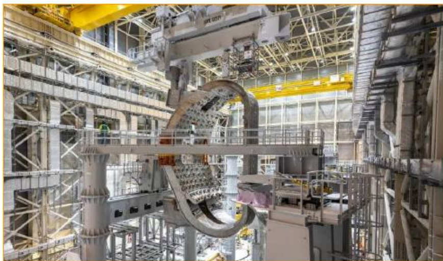
VVS6 lifted into the sector sub-assembly tool (SSAT)
