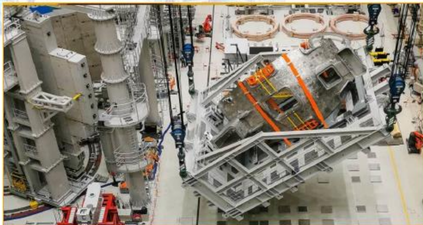
Up-ending VV Sector 6 with special tool
